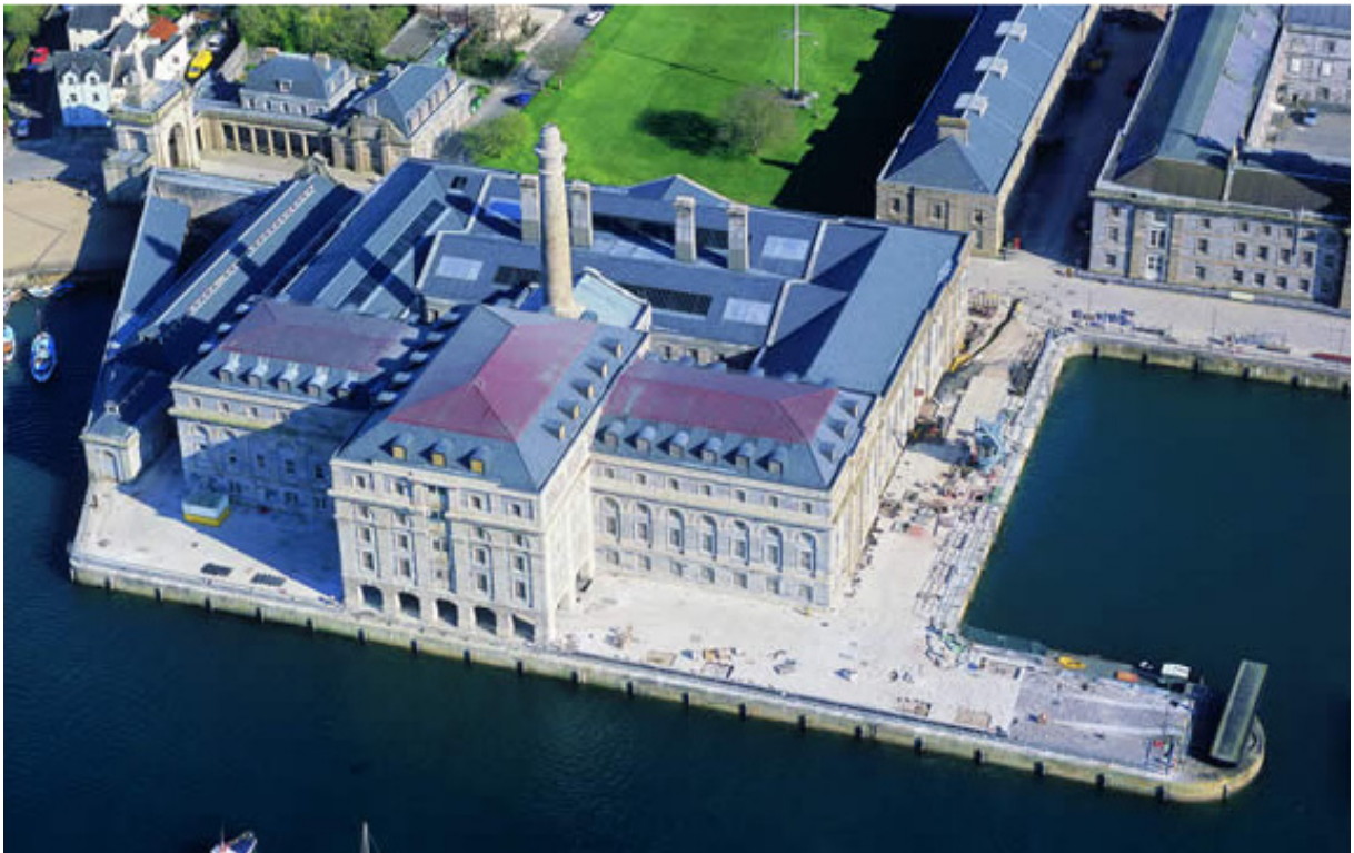
Image 5.19, Mills Bakery, Gillespie Yunnie. Seen as a key historical building, the mill required a new use to regain its former glory.
