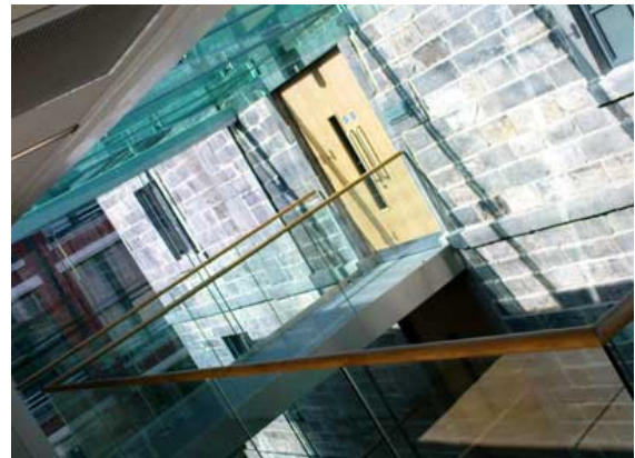
Image 5.27, Internal view which shows how the existing building has been adapted for change, the original delivery and work rooms have remained and been used for circulation. The old structure remains intact forming a successful working relationship with the new additions.
