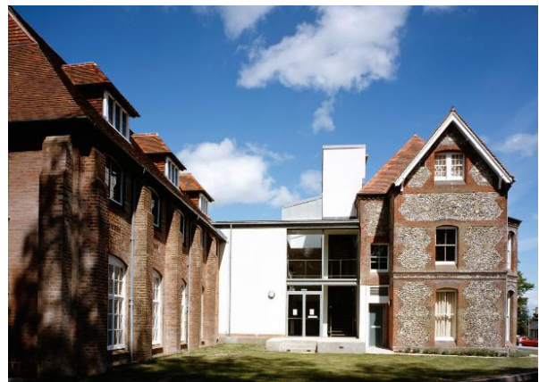
Image 5.24, External view showing both the retention of the existing building plus the additional modern interventions. The new additions don't take away from the existing structure, they are seen to add to its value and help create a sustainable new use.
