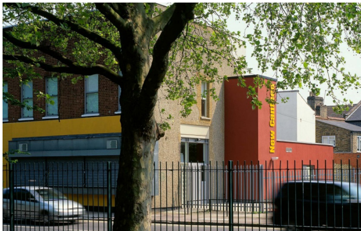
Image 5.14, Full external view, Emphasising how the simple additions and use of colour has completely brought life back to the area. Creating a building which the community can associate themselves with rather than be ashamed of was key.
